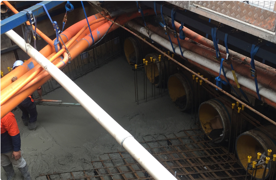
Top: Completed roof slab structure | Bottom Left: Reinforcing of base slab post completion of multiple parralel 820mm OD drives under road way | Bottom Right: Top view of civil works required for connection of services into basement separate to tunnelling works
