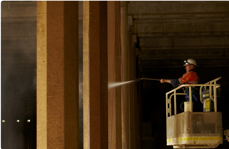
Top: Cleaning of silt inside reservoir | Bottom Left: Pressure cleaning reservoir internal columns using knuckle boom | Bottom Right: Applying the VOC free, fire resistant and UV stable VersEseal (spray grade) product to the reservoir roof.
