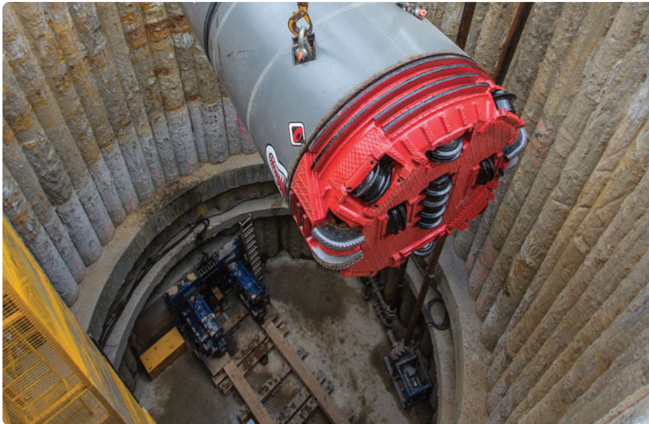
Top: Sweeping bend connecting piece for incoming lines installed and ready for GRP manhole connection | Bottom Left: Iseki TCS1800 'Emily Rose' getting lowered into the launch shaft | Bottom Right: Singular 16m long GRP manhole getting lowered into the shaft for connection into new pipeline.
