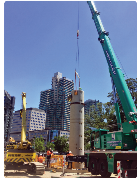
Top: Sweeping bend connecting piece for incoming lines installed and ready for GRP manhole connection | Bottom Left: Iseki TCS1800 'Emily Rose' getting lowered into the launch shaft | Bottom Right: Singular 16m long GRP manhole getting lowered into the shaft for connection into new pipeline.
