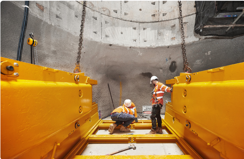
Top: 6 m ID segment caisson shaft to 23 m deep on Lonsdale Street | Bottom Left: Setting of jacking frame to launch shaft MTBM on Lonsdale Street | Bottom Right: 99th GRP Jacking Pipe being installed within launch shaft for first 550 m drive
