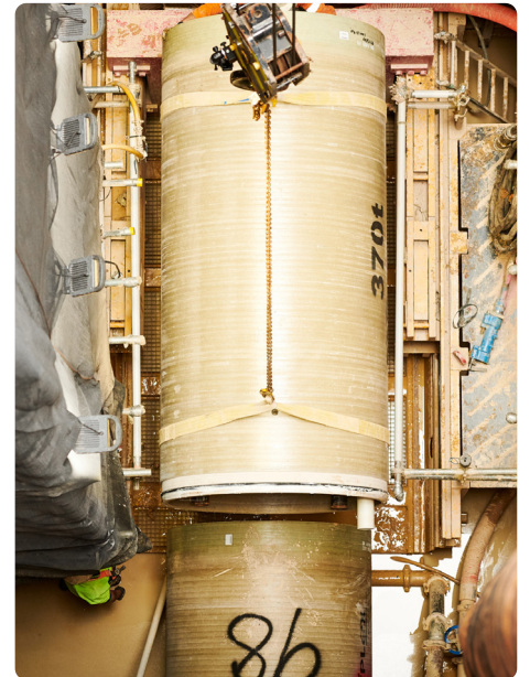
Top: 6 m ID segment caisson shaft to 23 m deep on Lonsdale Street | Bottom Left: Setting of jacking frame to launch shaft MTBM on Lonsdale Street | Bottom Right: 99th GRP Jacking Pipe being installed within launch shaft for first 550 m drive
