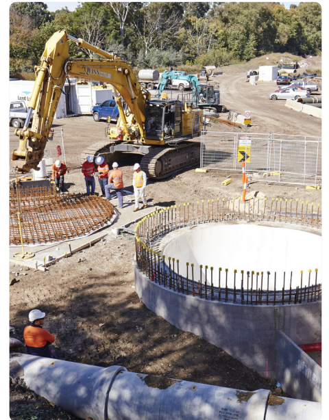
Top: Initial Launch of Iseki TCS1500 | Bottom Left: Iseki TCS1500 received at reception shaft | Bottom Right: Construction of DN5000 in situ concrete manhole
