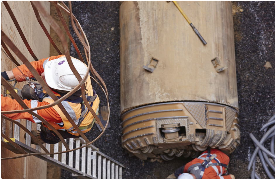
Top: Initial Launch of Iseki TCS1500 | Bottom Left: Iseki TCS1500 received at reception shaft | Bottom Right: Construction of DN5000 in situ concrete manhole
