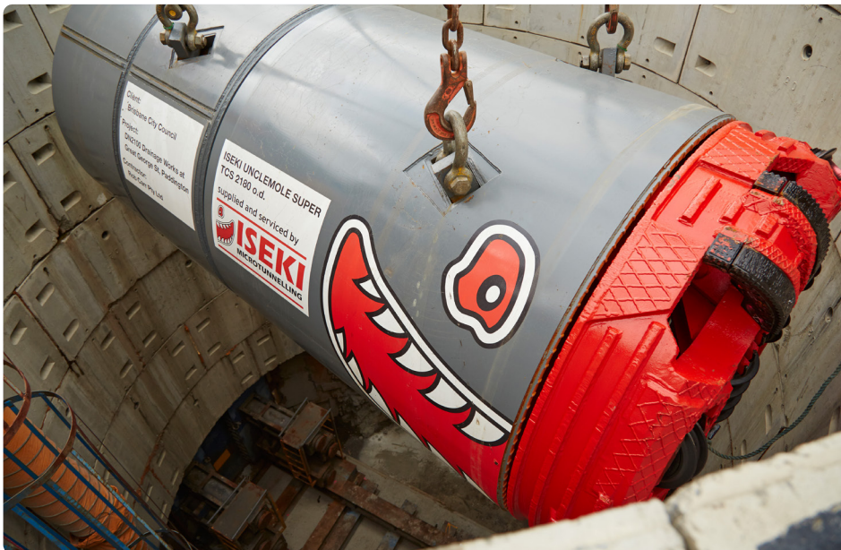
Top: The Iseki TCS1800 being transported along the suburban streets of Paddington in Brisbane QLD | Bottom Left: Lowering TCS1800 Unclemole Super into launch shaft | Bottom Right: 130T crane lifting the Iseki TCS1800 Unclemole Super off transport truck at launch site..
