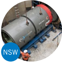
Microtunnelling & Civil Works Sub-Contract for Green Square Stormwater Drain Project
