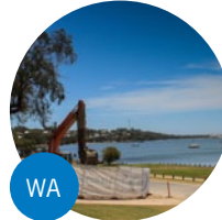
Dawesville 1B, 4A & 5A Infill Sewer Project
