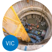
Metro Tunnel Early Works – Domain South Yarra Sewer
