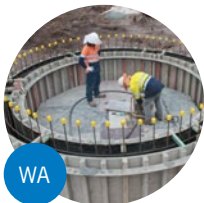
Busselton 18A & 12C Infill Sewer Project
